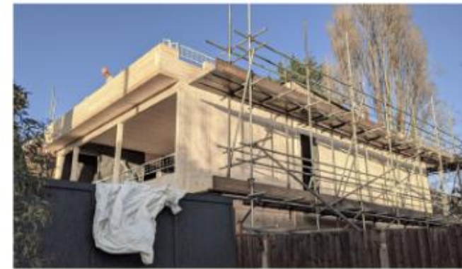
Delivering the CLT panels with weather protection membranes to the restricted site (top), and the CLT frame almost complete (below).
